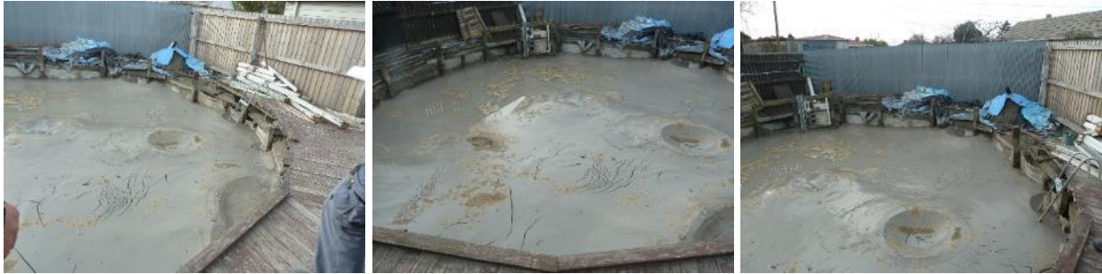
Figure 81: Ground photographs showing ejecta in the Swimming Pool (photograph date: 17 June 2011).
