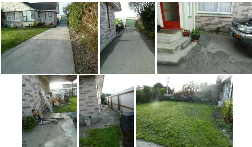
Figure 74: Ground photographs showing ejecta at the property with Patch A (photograph date: 17 June 2011).
